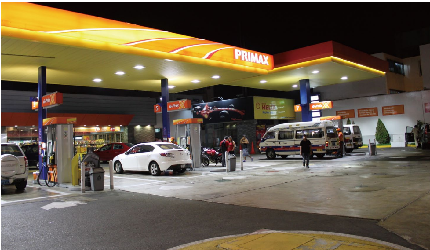
Primax Petrol Station, Peru
