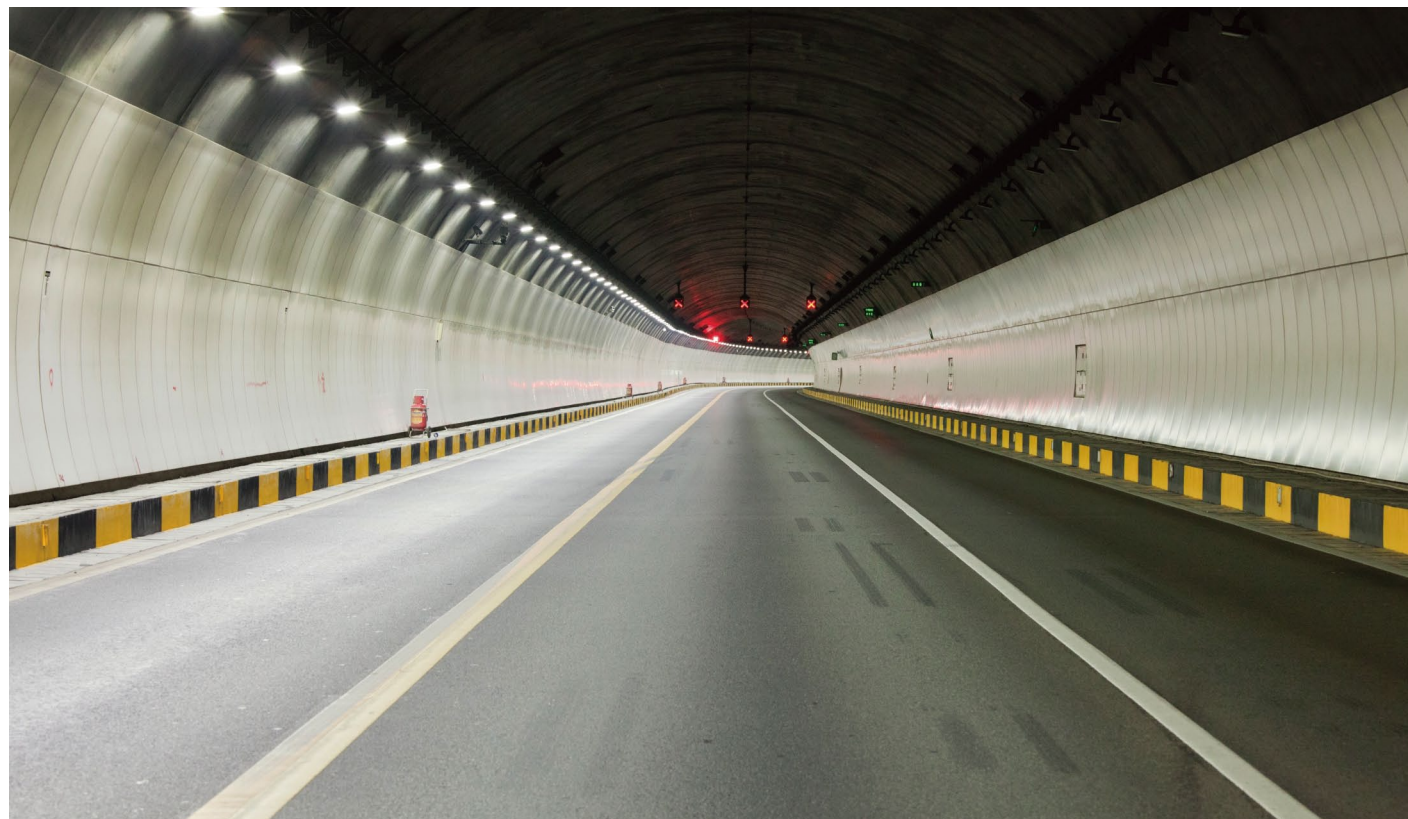
Shenzhen Highway, China
