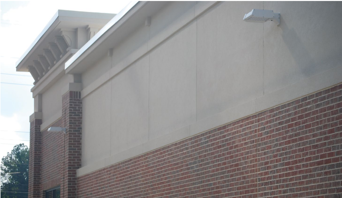
Richifield Building G.A. USA
