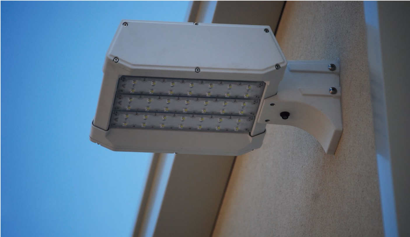
Richifield Building G.A. USA
