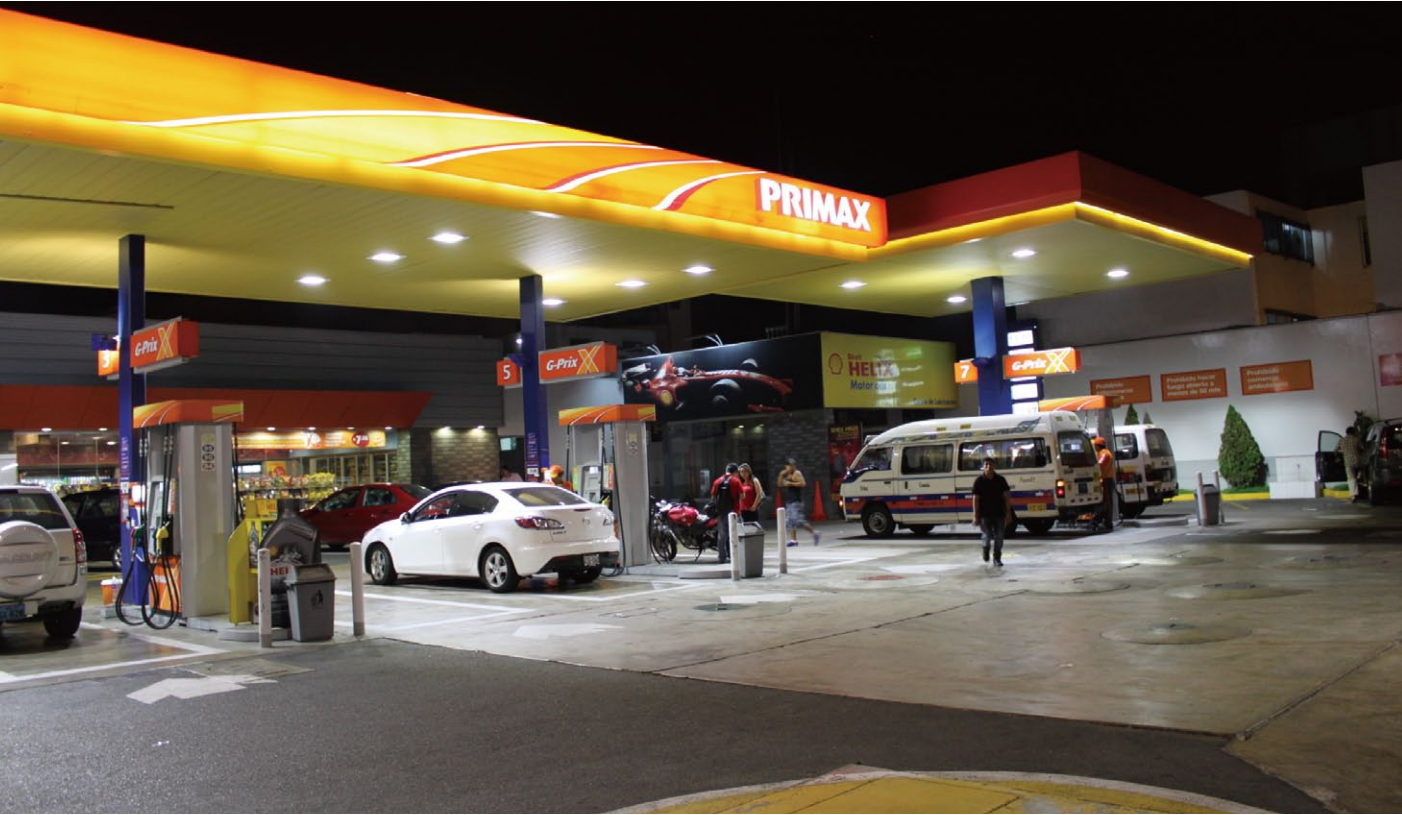
Primax Petrol Station, Peru
