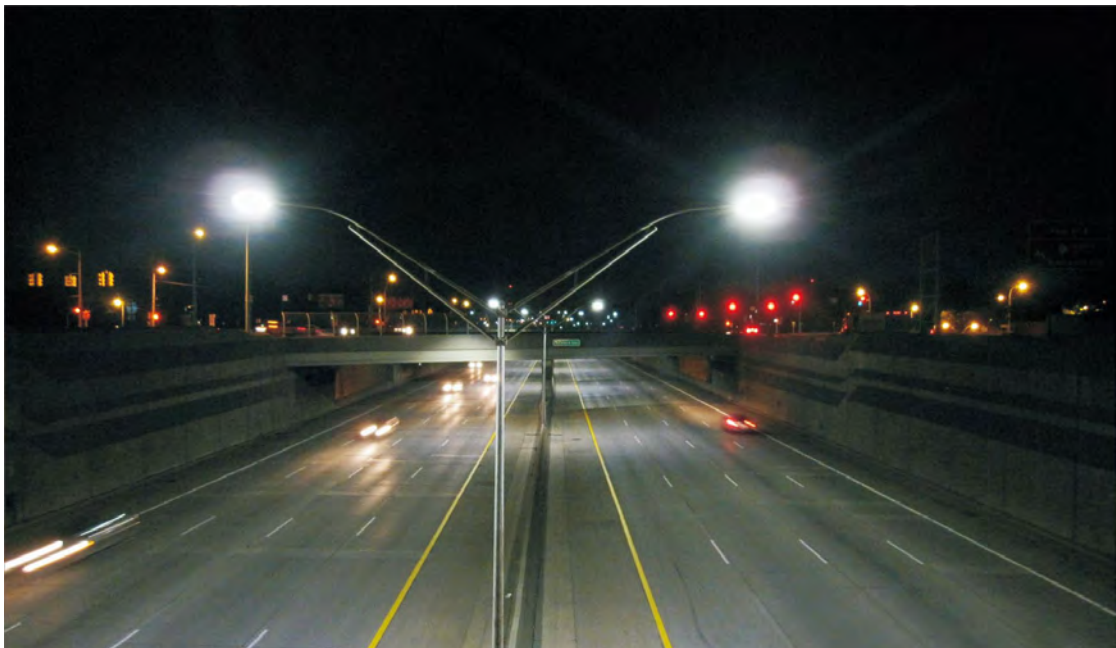
Highway LED Lighting Retrofit Project
