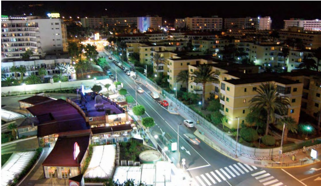
LED Lighting Retrofit Project
