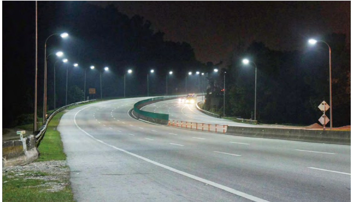
17-km roadways LED Lighting Retrofit Project
